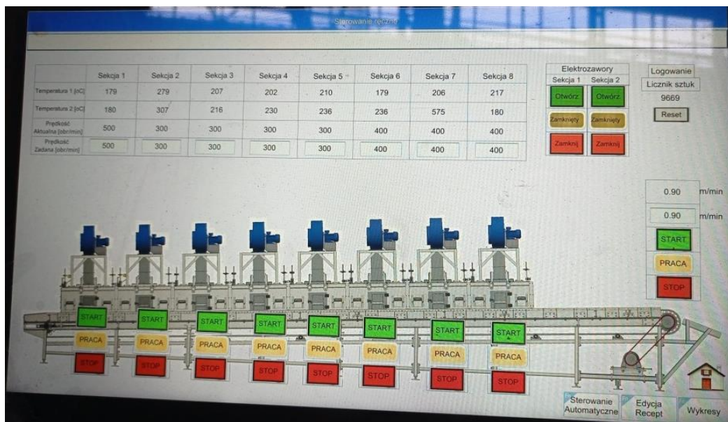
Fig. 7. Conveyor operation controller screen
