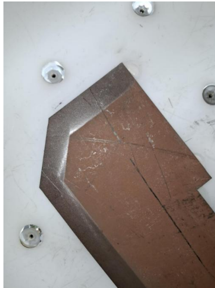
Fig. 9. Before/after photos showing part quality improvement
